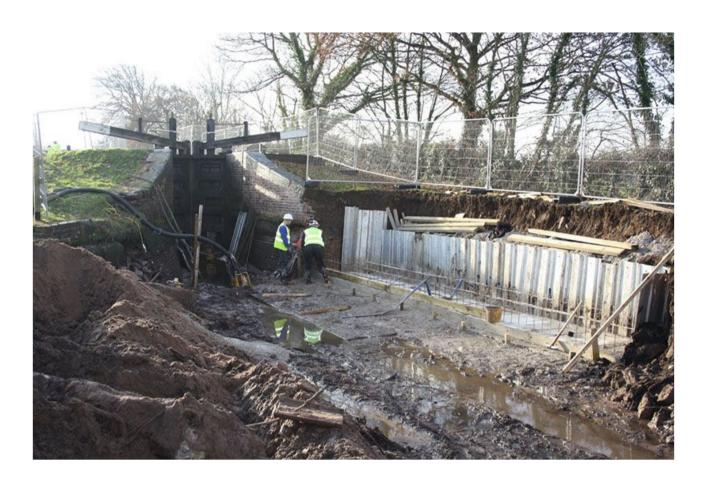
And at the landmark three lock staircase at Grindley Brook, each lock chamber is being improved with repairs to the gates, posts and chamber walls, including a new gate at the bottom.
