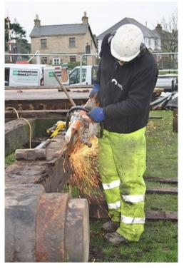
The wooden frames, which are made of the dense hardwood greenheart, have been in situ for at least 40 years and are amazingly still in good condition but the corroded metalwork and oak planking are being replaced.
