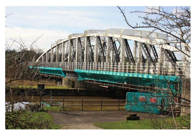
The work has been arranged by the Canal & River Trust, which cares for the River Weaver and 2,000 miles of the nation's waterways, and is being funded by Cheshire West and Chester Council. The work involves a complete refurbishment of the bridge deck, including strengthening to its underside, as well as improvements to the bridge appearance.
