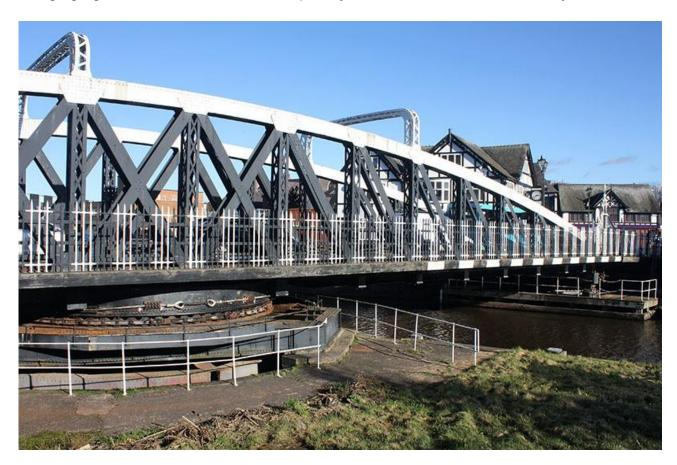
The waterways and wellbeing charity, which cares for the grade two listed bridge and 2,000 miles of waterways, has carried out vital repairs to re-balance the original cantilever rotary mechanism – enabling the 122-year-old bridge to swing open again for boats.
